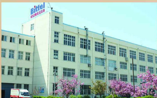
Outside view of workshop
